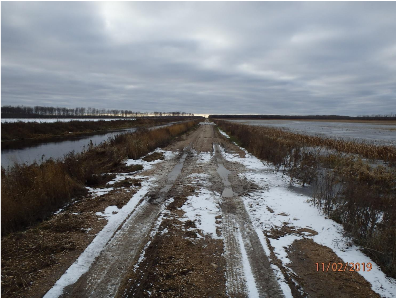
280 th St Looking West – Fall of 2019
