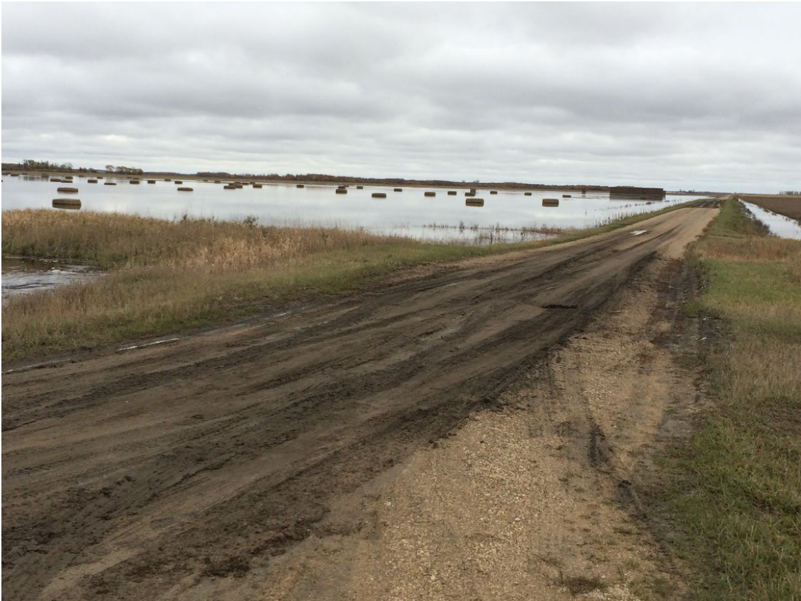
Looking SE at Section 6 Barto Twp – photo taken from NW corner of the section. Diversion will extend 4 miles south from here Diversion 160 th Ave
