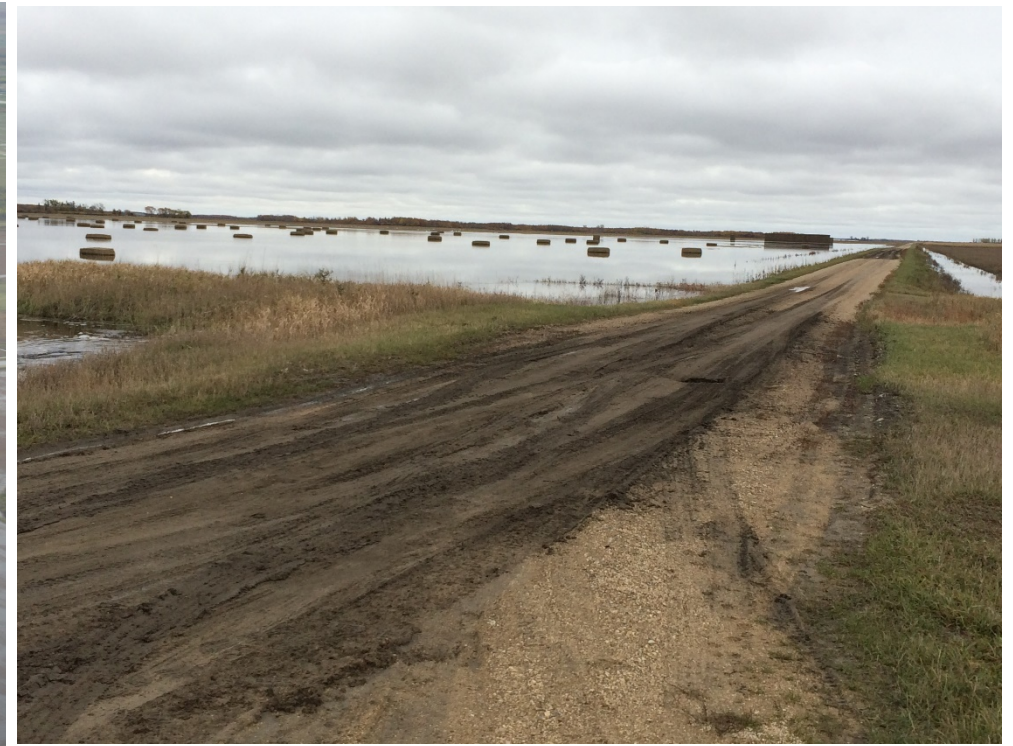
Looking SE at Section 6 Barto Twp – photo taken from NW corner of the section. Diversion will extend 4 miles south from this location
