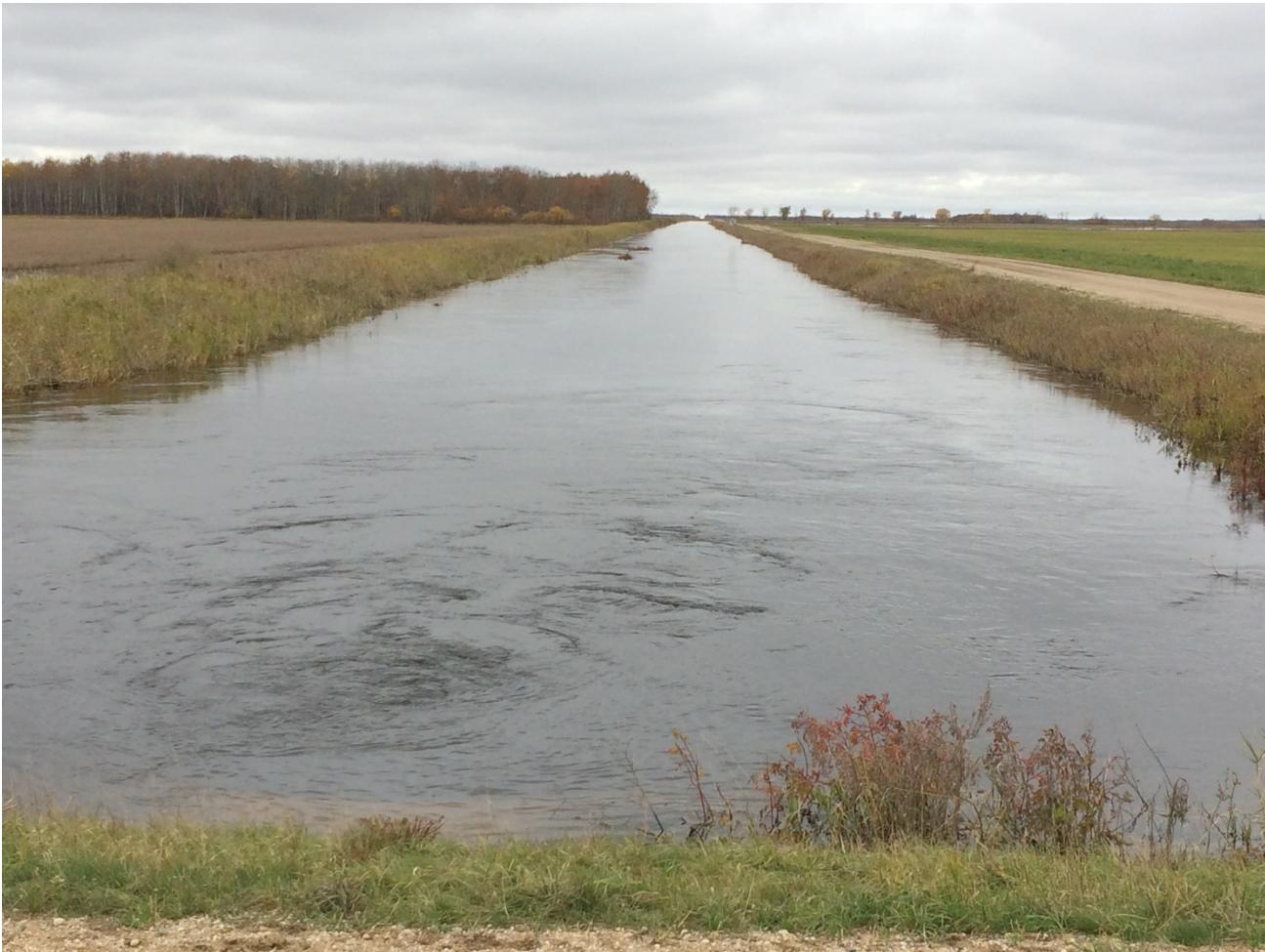
Lat1 SD95 at Roseau County Road 103 – looking west The 'New' 95 will be located on the south (left in this photo) side of the existing ditch
