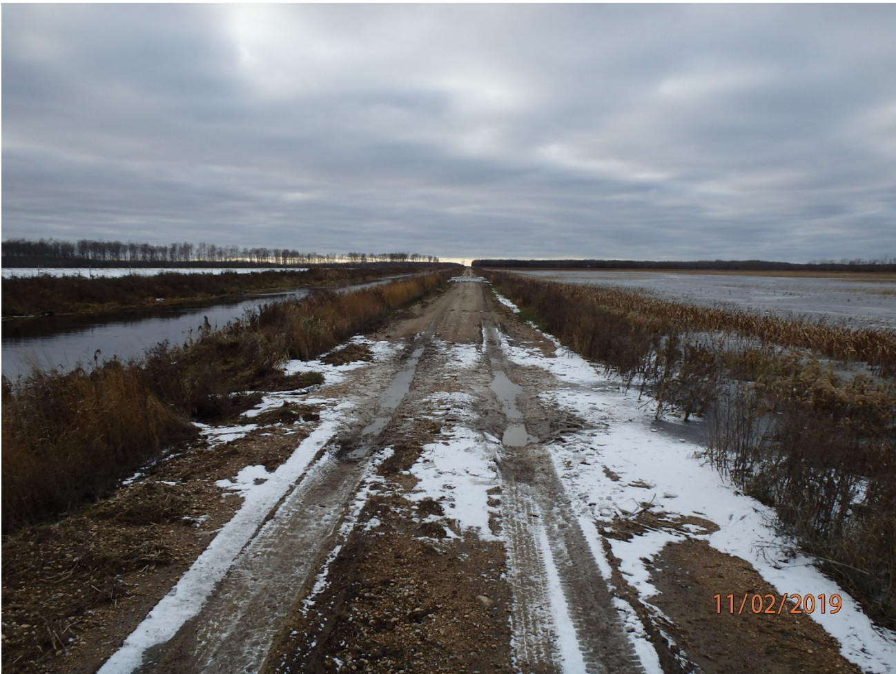
280 th St Looking West – Fall of 2019
